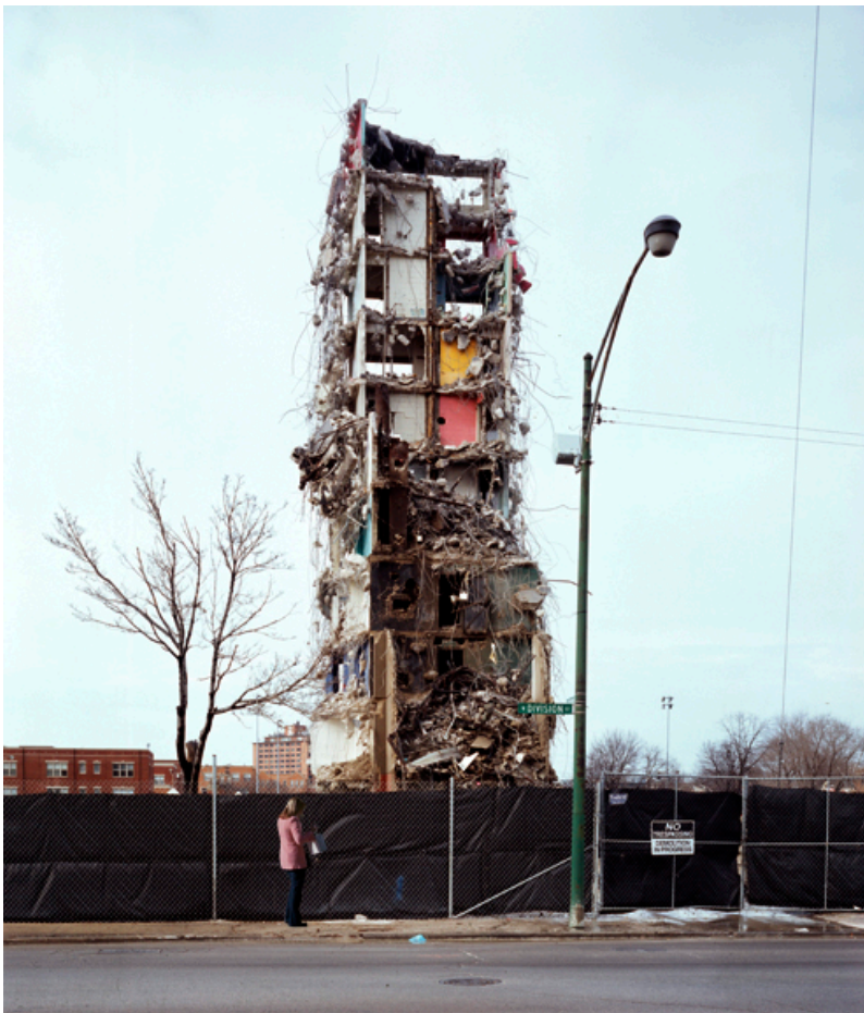
Figure 9. Cabrini Green housing project tower block under demolition, circa 2006. (Photographer unknown 10 .)
