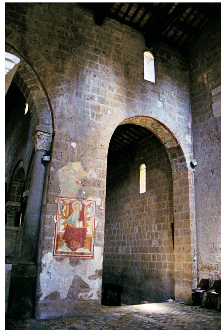
Fig. 15. Sant'Elia, north transept, west wall, including south transept pier. (Photo: author).
