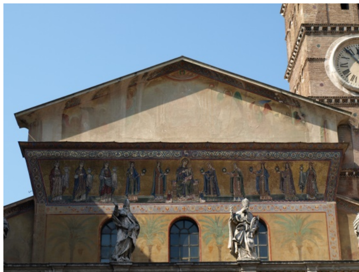
Fig. 6. Detail of façade. Photo: author.
