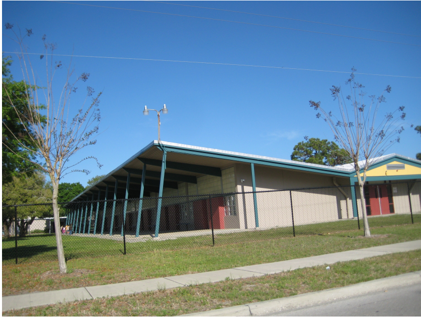
Image 6: Alta Vista Elementary School Addition, main façade, looking north, April 2010.
