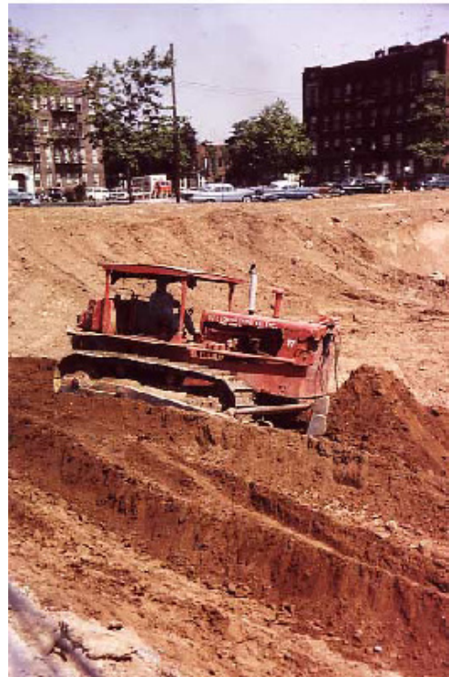
Figure 10. A Gull Contracting Co. vehicle shovels earth in Bay Ridge to make way for the Verrazano-Narrows Bridge. Source: Walsh 2003
