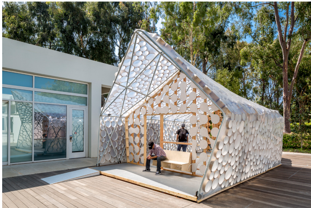
Figure 1. BI(h)OME ADU designed by Kevin Daly Architects. Concept by Dr. Dana Cuff. Image courtesy of UCLA cityLAB. Image credits: Nico Marques/Photekt.
