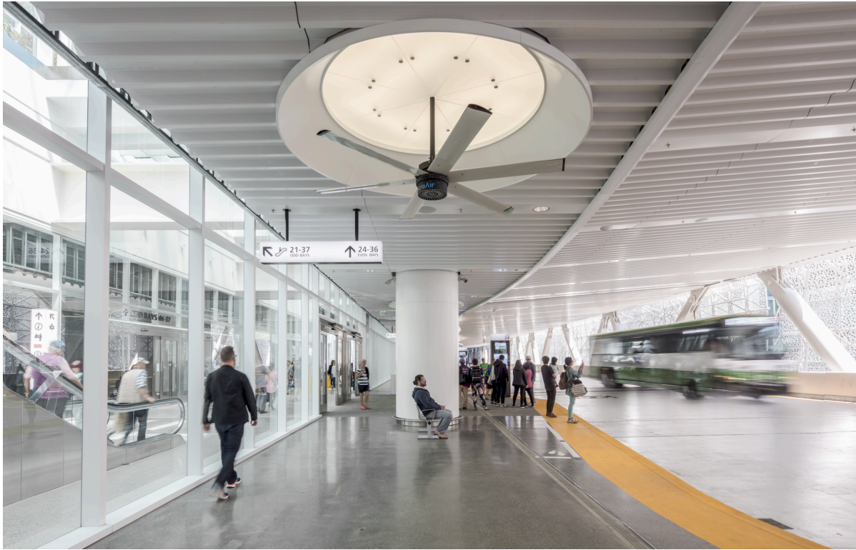
Figure 9: A photograph of the interior of the Salesforce Transit Center in San Francisco, designed by Pelli Clarke & Partners (architect), Peter Walker Partners (landscape architect), with consulting by Chris Downey. Photograph shows a glass window wall and polished grey concrete floor with a metal tactile strip or groove set into the surface next to a wide, yellow painted stripe at the bus port. Image courtesy of Jason O’Rear.
