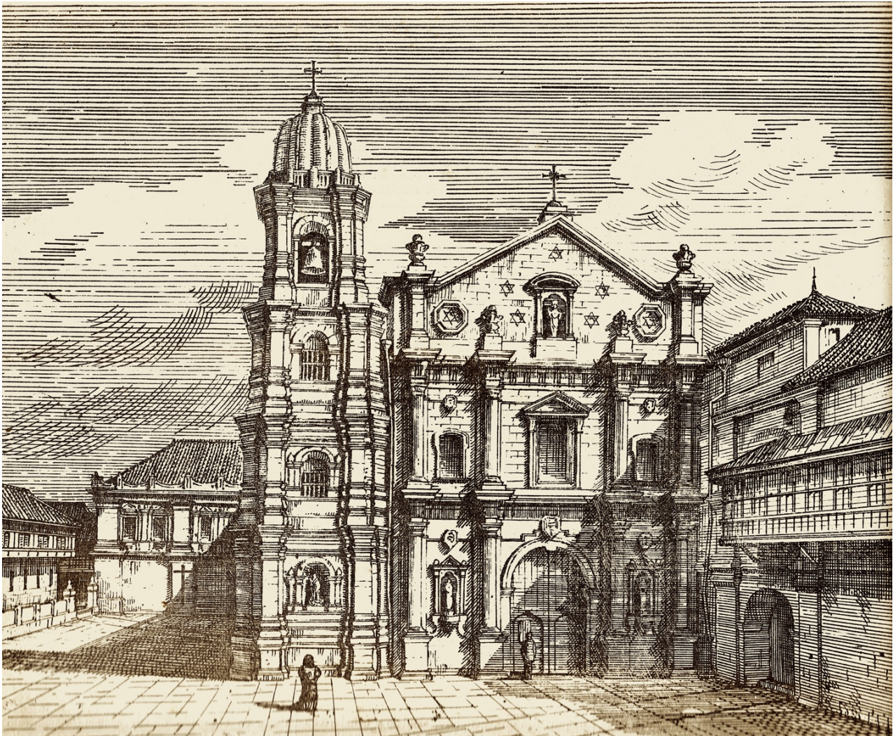
Plate 4. Saint Francis of Assisi Church, Manila, El Oriente , 31 July 1875.
