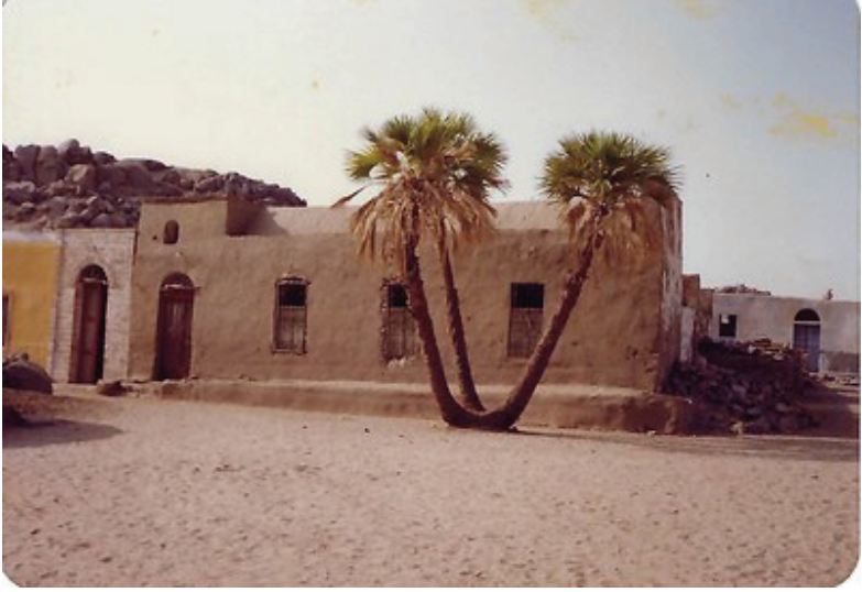
Figure 5. Most houses have benches of smoothly plastered clay ( mastabas ) that are built along the fronts of the outside walls. (Jennings, 1981).
