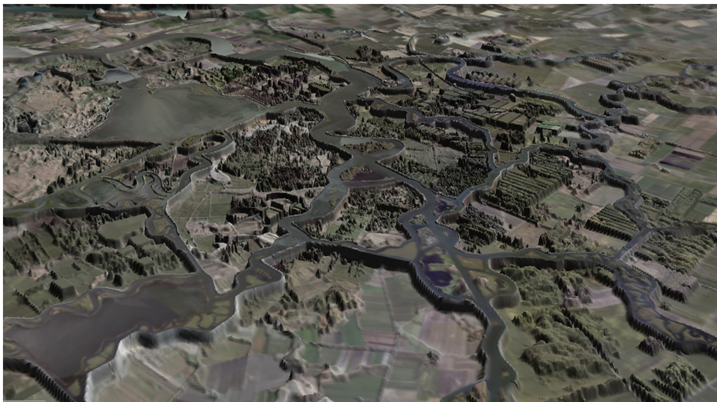
Figure 1 Poldered islands in the Sacramento-San Joaquin Delta, viewed as a digital elevation model overlain with satellite imagery and with vertical relief exaggerated 10x. Two large permanently flooded polders are shown on the left half of the image. The other tracts range from 3-8 meters below sea level. Irregularities in polder surfaces are due to orchard crops, dikes, and buildings (Image credit: Burak Yikilmaz).
