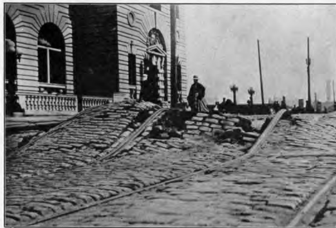
RESULT OF EARTHQUAKE on street and car tracks in front of Postoffice.
