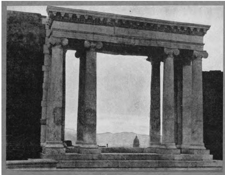
Fig. 49: Louis J. Stellman's photograph of the former entrance to the Towne Mansion, which has become famous as the 'Portals of the Past.' (F869.S3.93.S8: 16-17). From Stellman's The Vanished Ruin Era (1910). Courtesy of the Bancroft Library, University of California, Berkeley.
