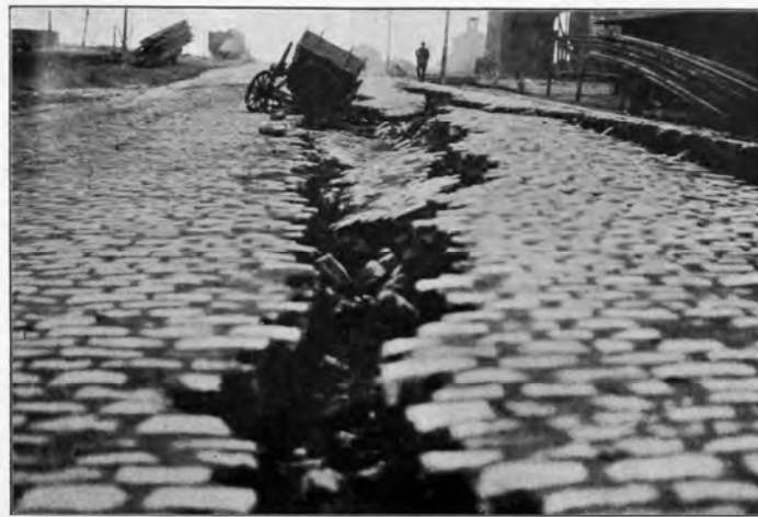
EFFECT OF THE EARTHQUAKE ON EAST STREET.
