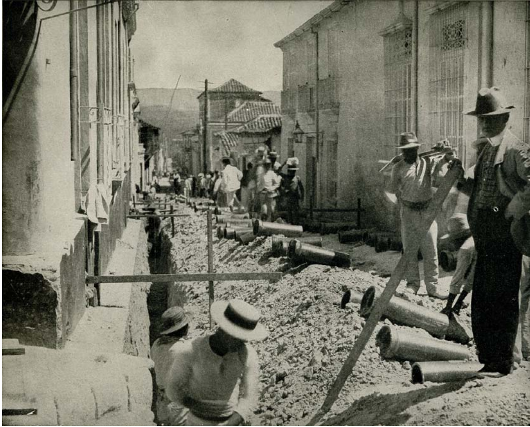
“Laying Drain Pipes in Santiago,” from Olívares’s Our Islands and Their Peoples (1899).
