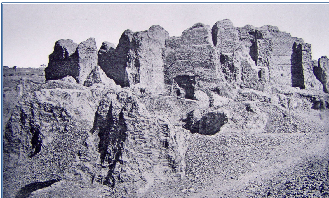
Figure 6. Remains of tower houses in Bubastis in 1880.
