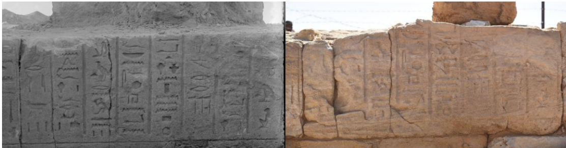
Figure 5. Photographs of a single section of the Sanam Historical Inscription, taken in both 1912 and 2018, demonstrating the temple's deterioration.
