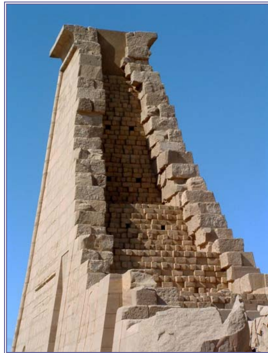
Figure 3. East tower of Horemheb's Ninth Pylon, Karnak. The interior core is composed of much smaller talatat blocks from Akhenaten's monuments at Karnak.
