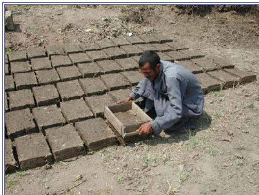
Figure 1. Unmolding new mud-brick.
