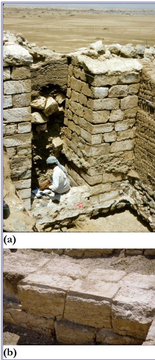
Figure 5. Examples of structures built with anhydrite and gypsum: a) gypsum gate in wall of Abu Sha'ar fortress (late Roman Period; near Hurghada [el-Ghardaqa]); b) anhydrite and gypsum ashlar at Marsa Nakari, the putative ancient Nechesia (early Roman Period; near Marsa Alum).
