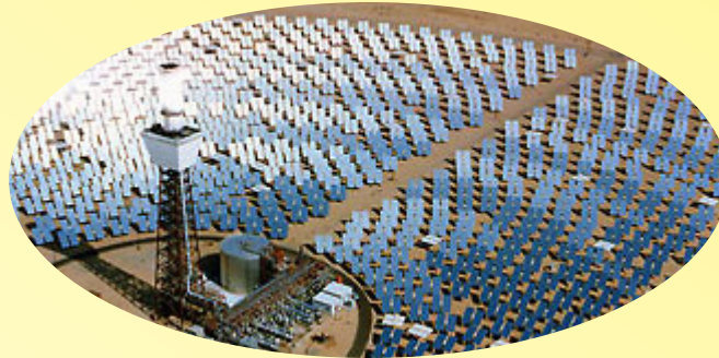
Solar Two was a proof-of-concept solar-thermal energy plant that used molten salt to capture and store the sun's heat, allowing for energy production even at night.
