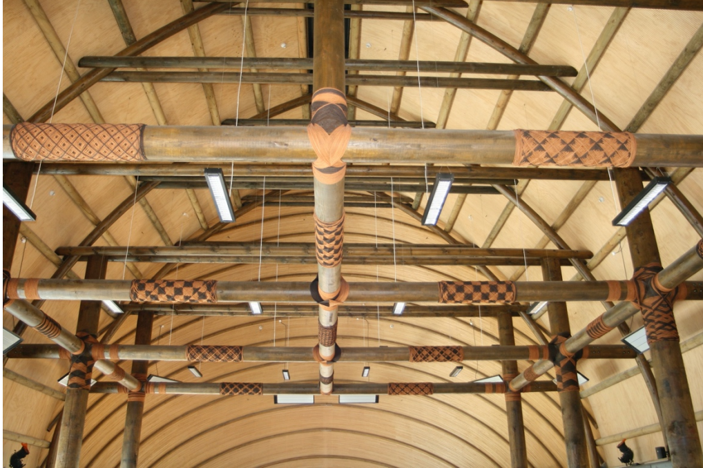
Figure 2. Sopolemalama Filipe Tohi , lalava made with kafa (sennit) lashing. Fale Pasifika, Auckland University, installed c. 2004. Photograph courtesy of Hilary Scothorn
