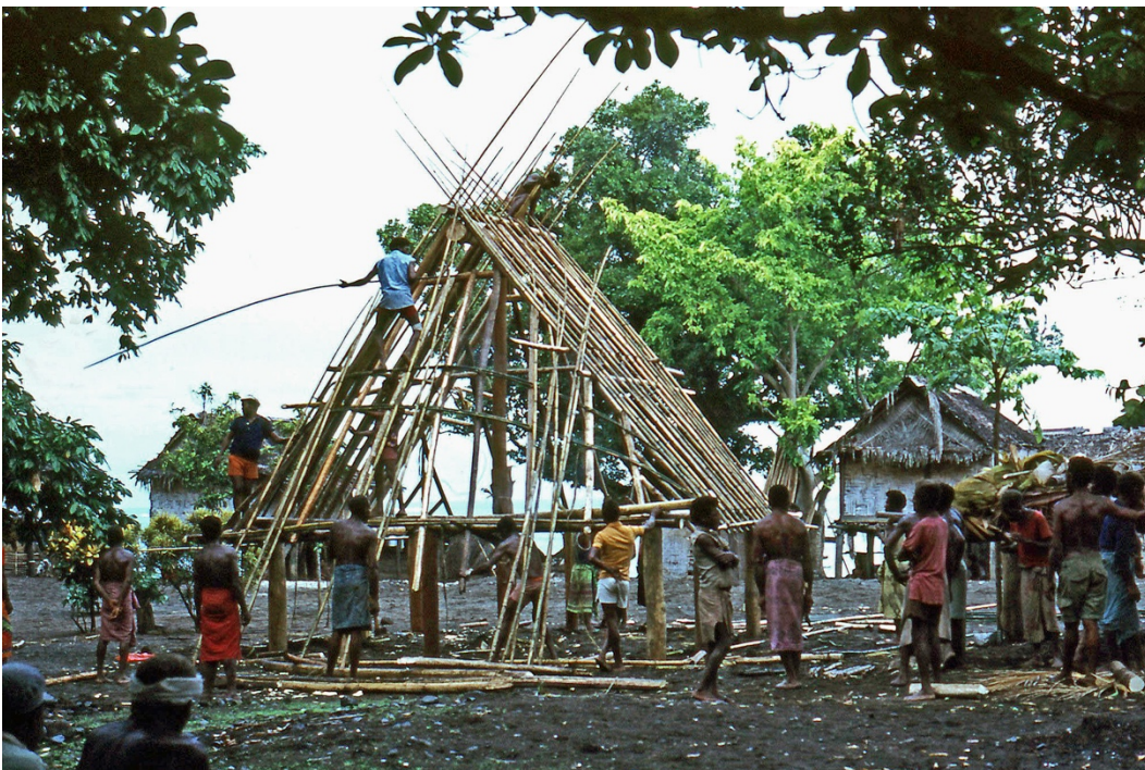
Figure 23. Construction of the naulum roof. Potne village, Kilenge, West New Britain, Papua New Guinea, c. 1977. Photograph courtesy of the author
