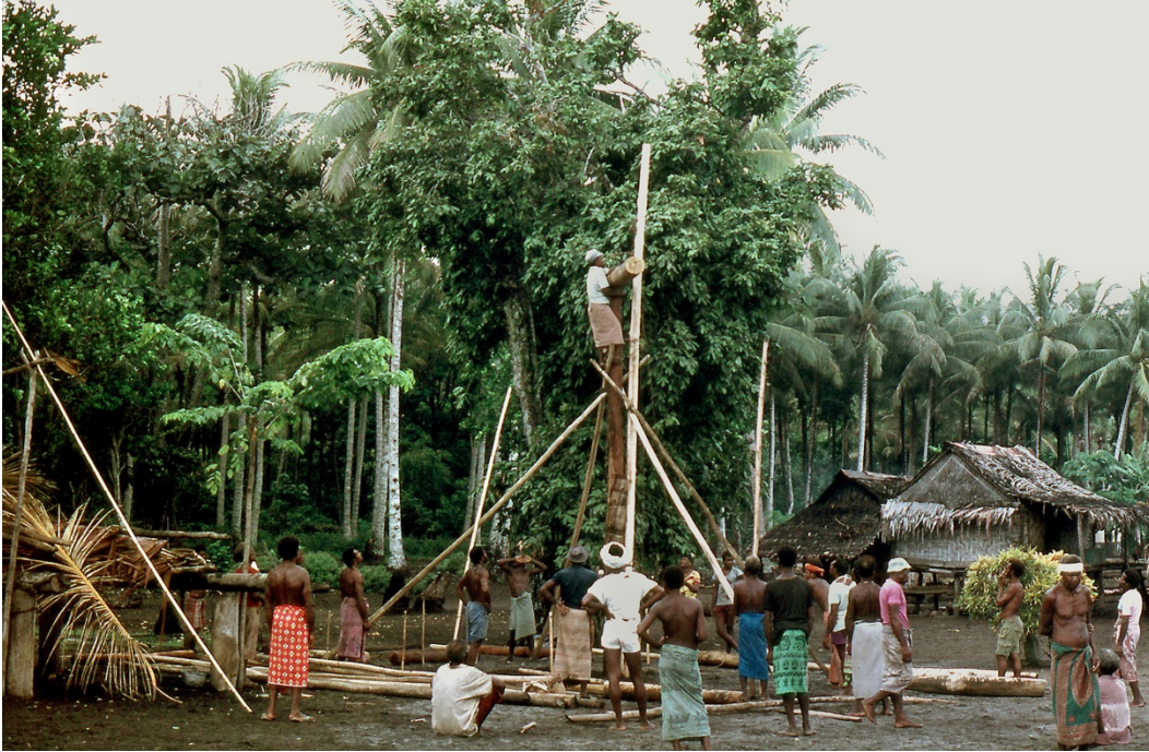
Figure 22. Construction of the naulum. Potne village, Kilenge, West New Britain, Papua New Guinea, c. 1977. Photograph courtesy of the author
