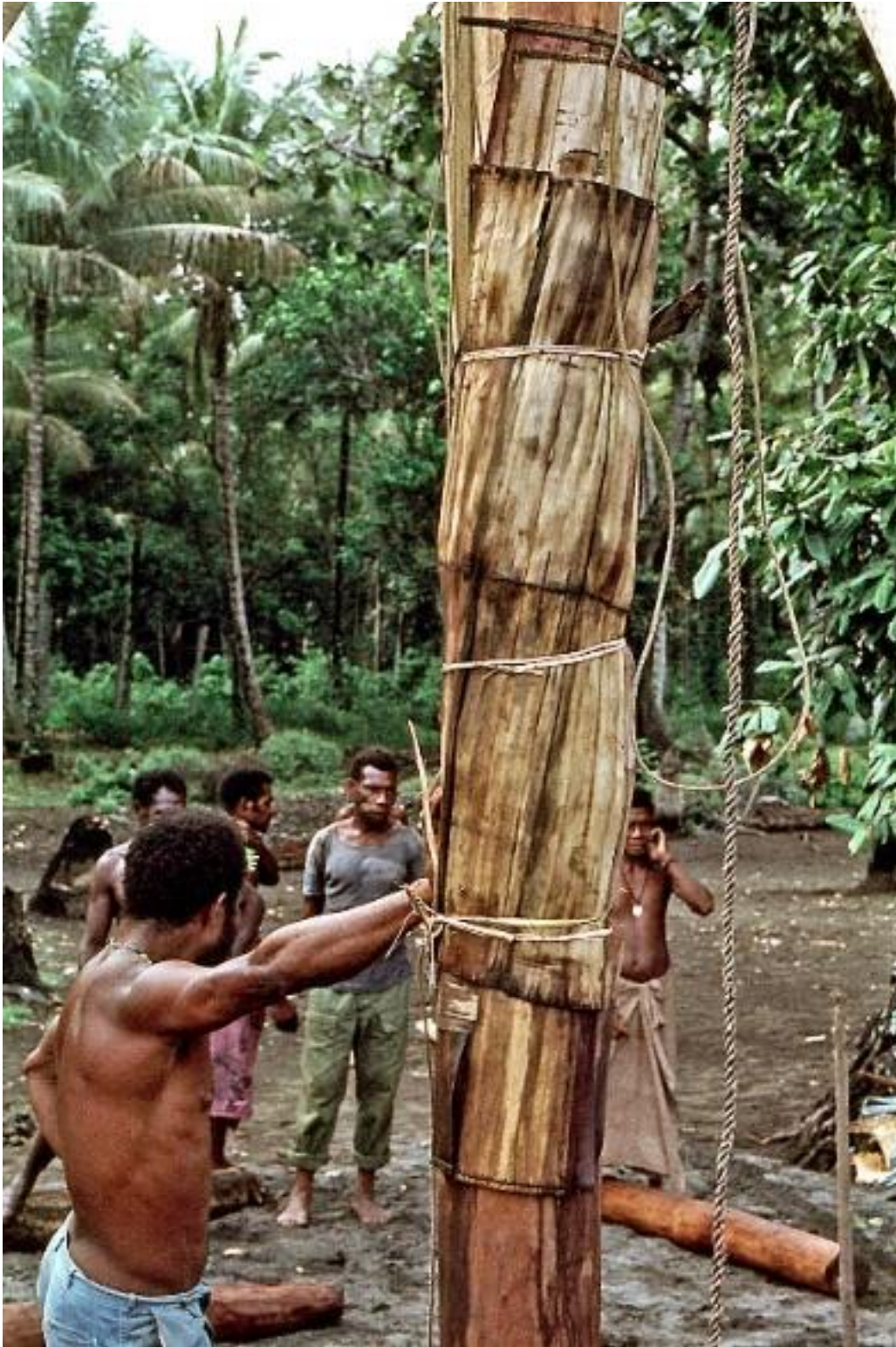
Figure 21. The central pole of the naulum is erected with the Nausang face still protected by leaves. Potne village, Kilenge, New Britain, Papua New Guinea, c. 1977. Photograph courtesy of the author
