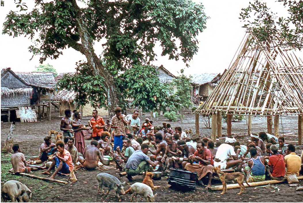
Figure 26. Having completed their work on the naulum for the day, the builders enjoy a meal sponsored by the local big man and prepared by Potne women. Potne village, Kilenge, West New Britain, Papua New Guinea, c. 1977. Photograph courtesy of the author
