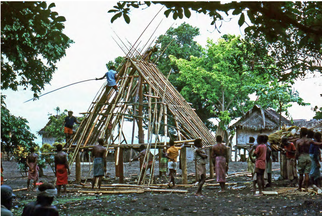
Figure 23. Construction of the naulum roof. Potne village, Kilenge, West New Britain, Papua New Guinea, c. 1977. Photograph courtesy of the author
