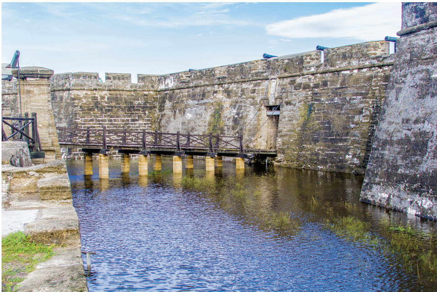
FIGURE 4. The Castillo de San Marcos is the oldest fortification in the United States, constructed between 1672 and 1695. Now under the management of the National Park Service as a national monument, it hosts about 850,000 visitors annually. The native coquina stone structure is vulnerable to sea-level rise, and the porous ground in Florida exacerbates threats. Photo courtesy Gary LeVeille, “Castillo de San Marcos National Monument flooding during Hurricane Matthew,” October 2016.
