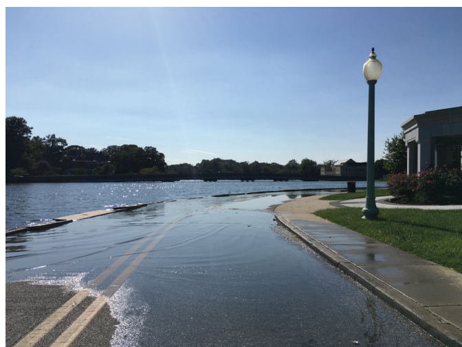
FIGURE 2. United States Naval Academy sunny day flooding: Ramsey Road on September 20, 2017, during high tide. The road frequently floods and has to be closed by security. This impacts memorial ceremonies and internments at the Columbarium, as well as impeding traffic to and from the faculty parking lots on Hospital Point. Historic Hubbard Hall is in the background. Photo courtesy Dr. Angela Schedel, USNA alumnus.
