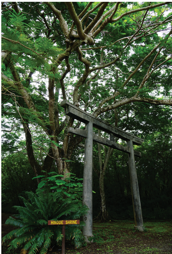
FIGURE 3. Participants in the vulnerability assessment training on Tinian identified a Torii (gate), part of a Japanese Shinto shrine built in 1941, as highly vulnerable due to the potential for the large adjacent flame tree to fall during a typhoon. The limited capacity of the CNMI Historic Preservation Office to perform vegetation maintenance was also identified as contributing to vulnerability. Two months after the assessment, category 5 Typhoon Yutu struck Tinian with wind gusts approaching 200 miles per hour. The flame tree in the photo came down in the storm, causing the Torii to collapse.
