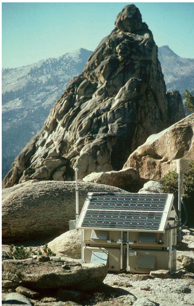
Solar-powered meteorological station at Emerald Lake.
