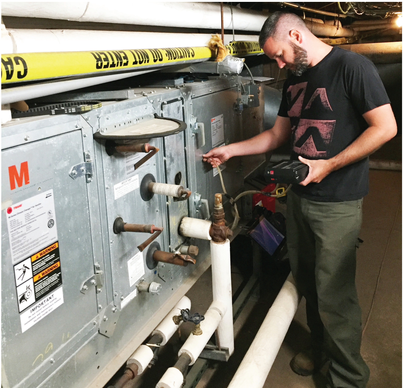
FIGURE 10 (above). Thermal imaging at Sagamore Hill. STEVEN WEINTRAUB, ART PRESERVATION SERVICES
