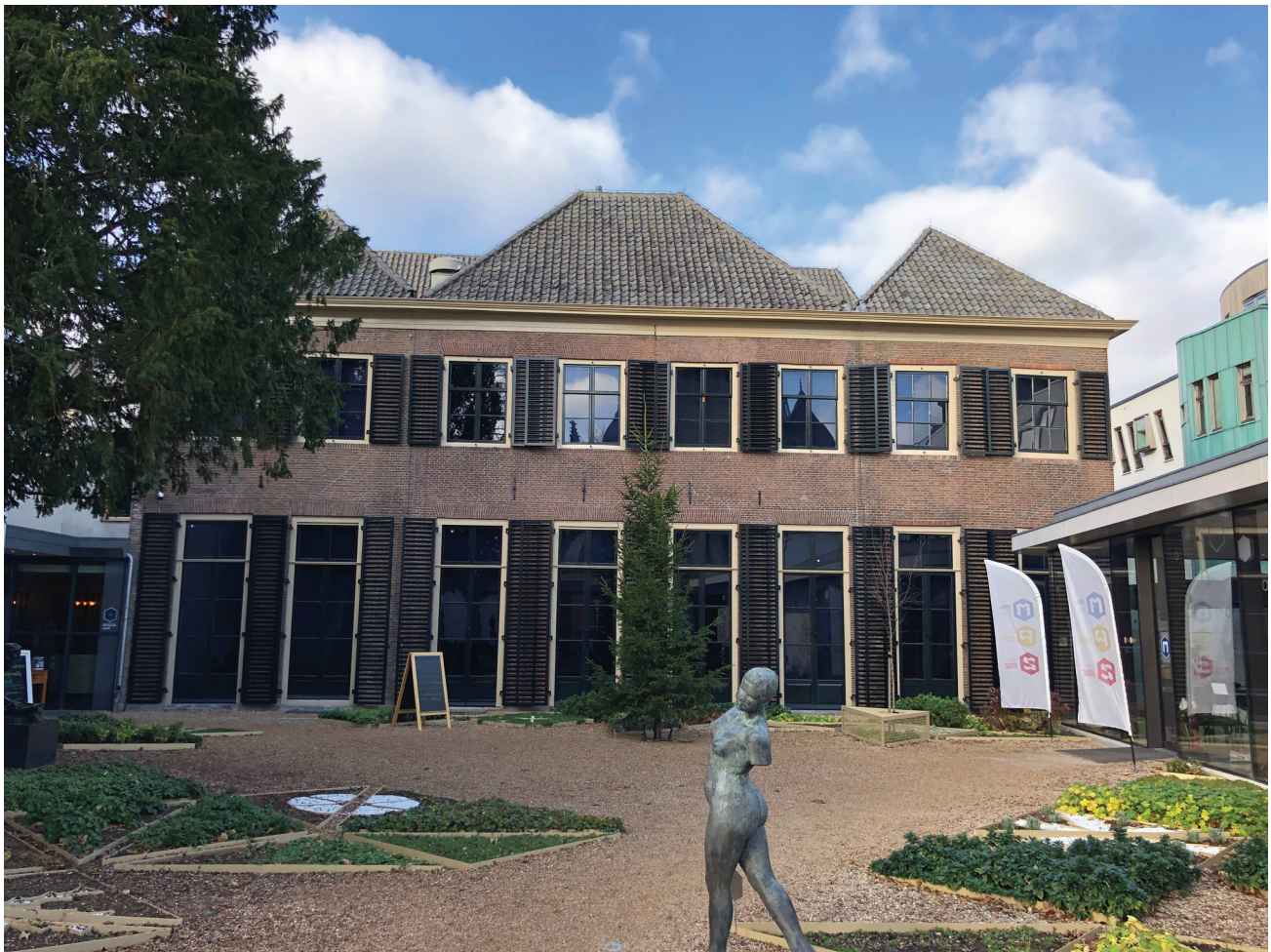
IMAGE 17. The exterior of Hof van Heeckeren in Zutphen with the new entrance on the right. Originally this side was the backside of the building. MARC STAPPERS
