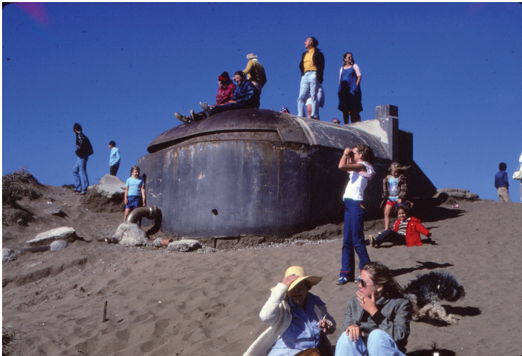
↓ Before and after viewing platform construction. LEFT: ROLF DIAMANT • RIGHT: CREATIVE COMMONS
