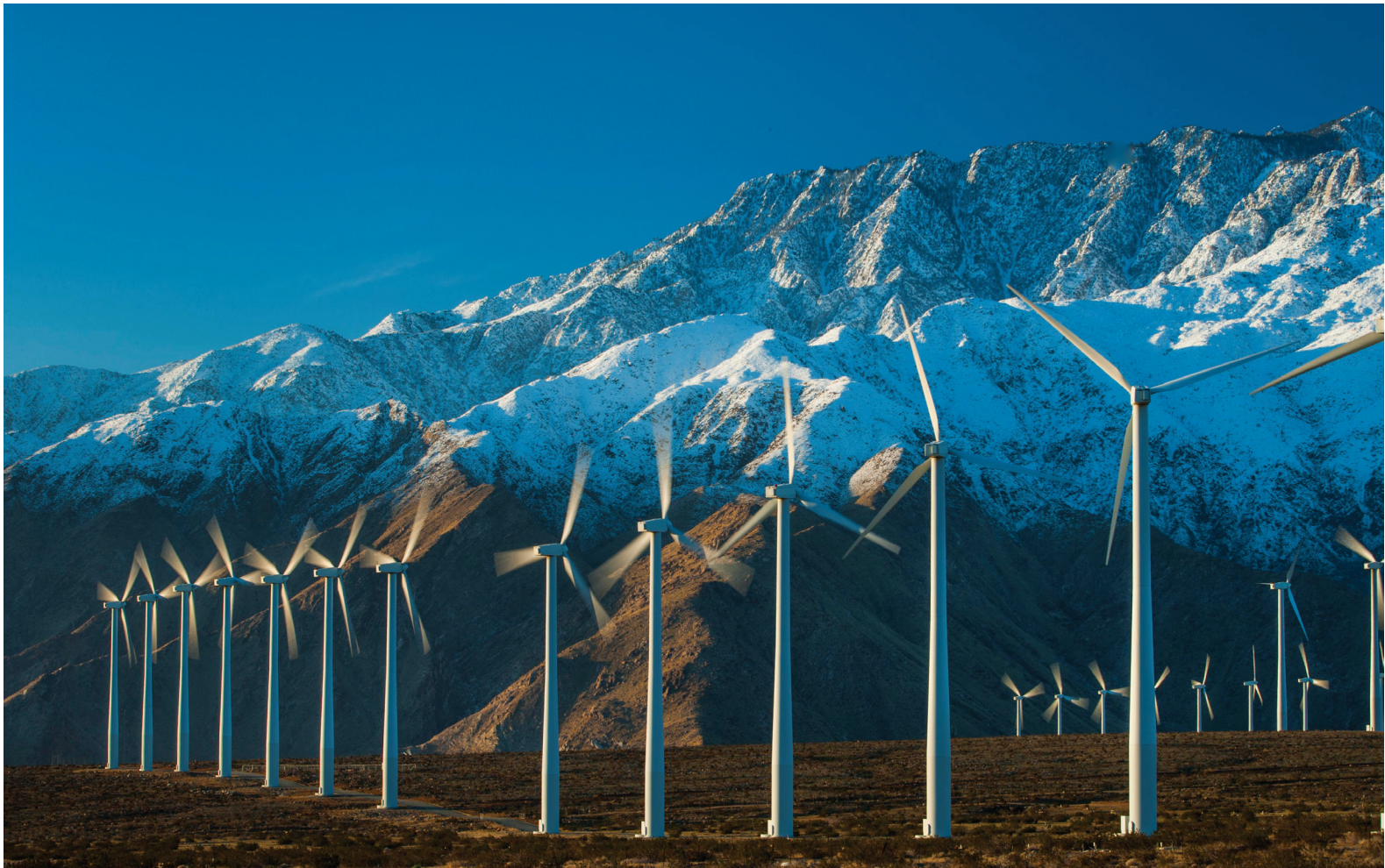
Santa Rosa and San Jacinto Mountains National Monument rises behind wind energy development north of Palm Springs California. Integrated planning for energy infrastructure and conservation outcomes is the goal for the Desert Renewable Energy and Conservation Plan. TOM BREWSTER, BLM
