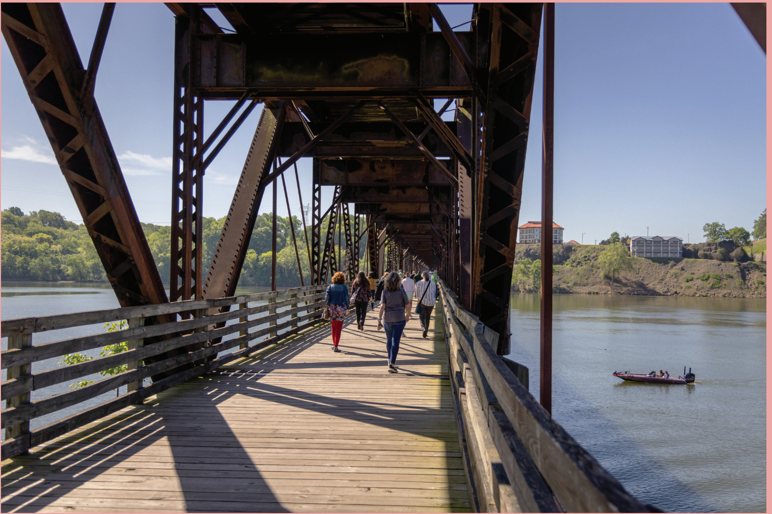
Memphis & Charleston Railroad Bridge. ABRAHAM ROWE
