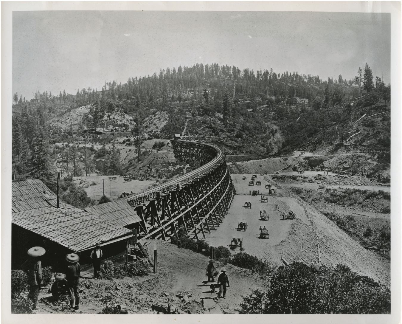
Chinese railroad workers in the Sierra Nevada Mountains (Placer County, California), ca. 1877. They are likely performing maintenance and repair work on the original transcontinental line. SC3628, NORTHEASTERN CALIFORNIA HISTORIC PHOTOGRAPH COLLECTION, MERIAM LIBRARY SPECIAL COLLECTIONS, CALIFORNIA STATE UNIVERSITY, CHICO
