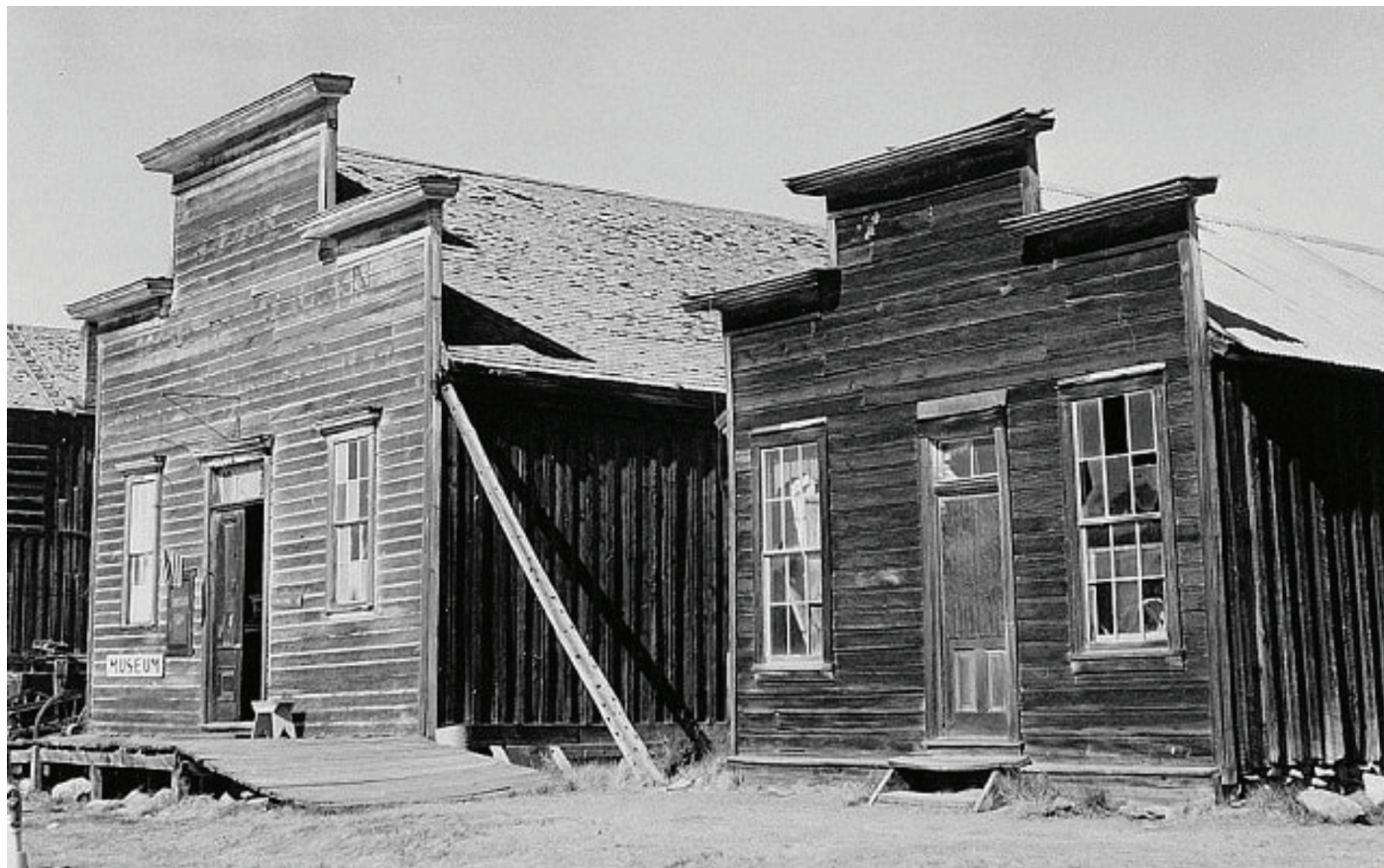
FIGURE 1. Miners’ Union Hall, Main Street, Bodie, California, ca. 1930s. LIBRARY OF CONGRESS, HISTORIC AMERICAN BUILDING SURVEY
