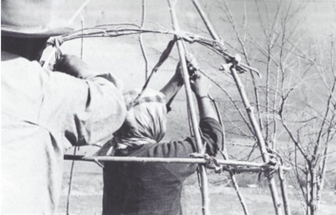
Figure 3: Jimmy George (left) and Daisy Aster (right) demonstrating traditional Northern Paiute shelter assembly with willow branches, 1967. Courtesy of University of Nevada Press.
