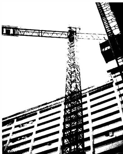
Figure 16: HDB Housing Being Upgraded
