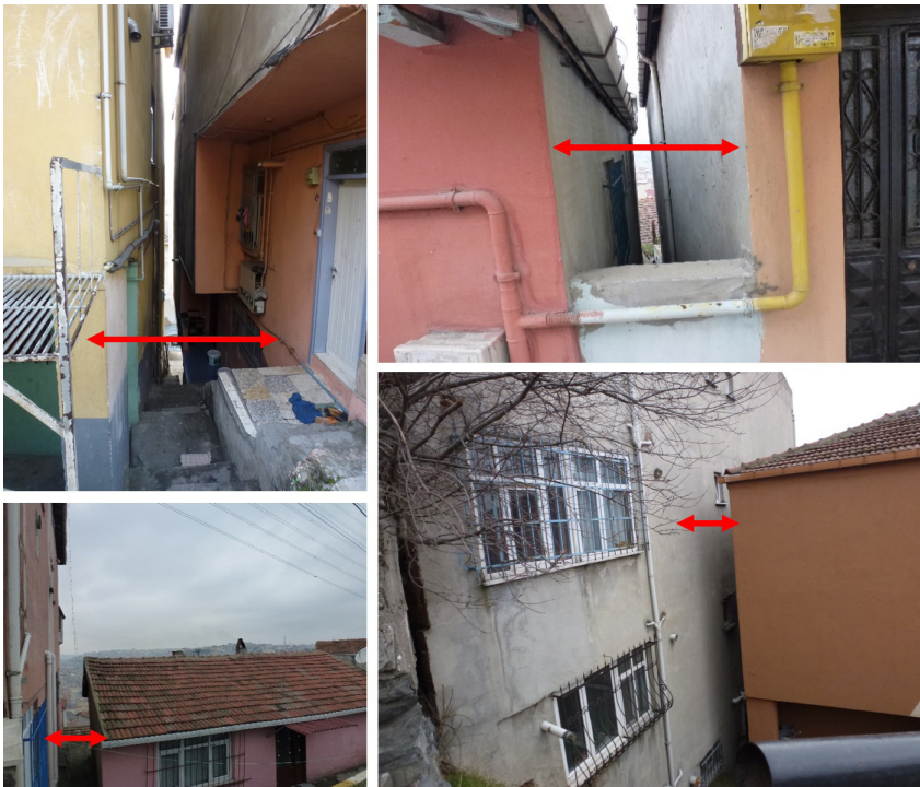
Figure 9 Gaps Between Buildings (Photo by the authors)
