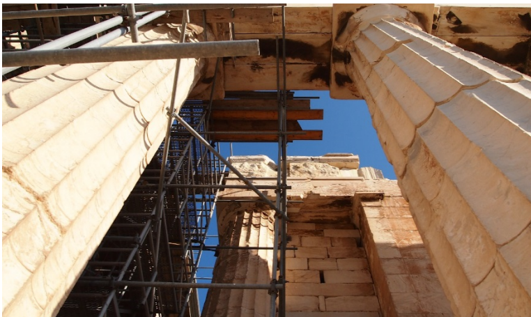
(2) View of the south-west corner of the Parthenon Ionic frieze, showing its situation over the architrave of the internal chamber and behind the exterior entablature. Photograph: Author.
