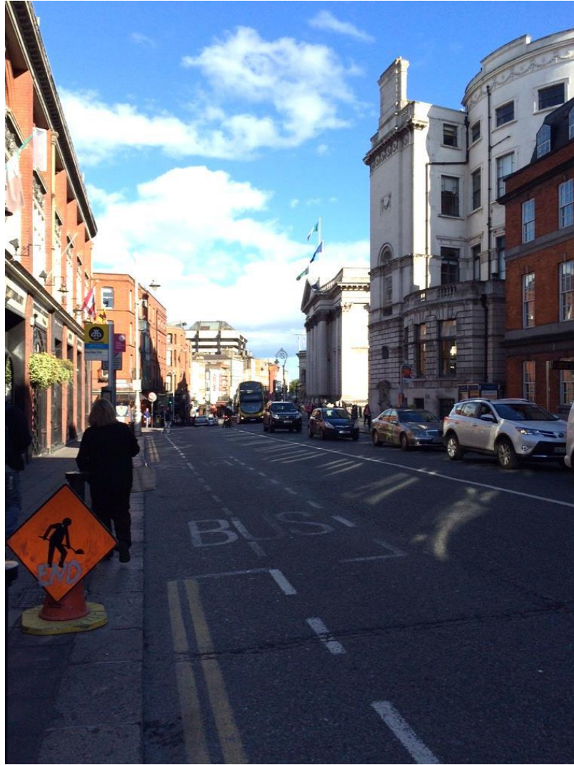
Fig. 1. View east, down Dame Street toward College Green. In the middle ground, at the right margin of the street stands Dublin City Hall. The tallest building depicted, the modern hipped-roof structure in the middle of the image, is the Central Bank of Ireland, 2016. Photo credit: S. L. Martin-McAuliffe.
