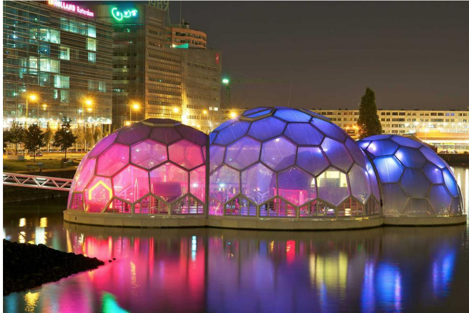
Fig. 5. The Floating Pavilion (2005-2010). Three interlinked spheres, the largest of which with a radius of 12 meters. The total floor space of pavilion island is 46 x 24 meters. An innovative and sustainable building, which is climate change resilient and reflects Rotterdam's adaptation strategy in response to climate change. Now that all commercial and industrial activity has been moved to massive transfer sites at the coast, the question remains of how to re-appropriate vacant former city harbors? Rotterdam's residents were previously so strongly connected to the harbor activities. How will they be involved with the waterfront in the future?
