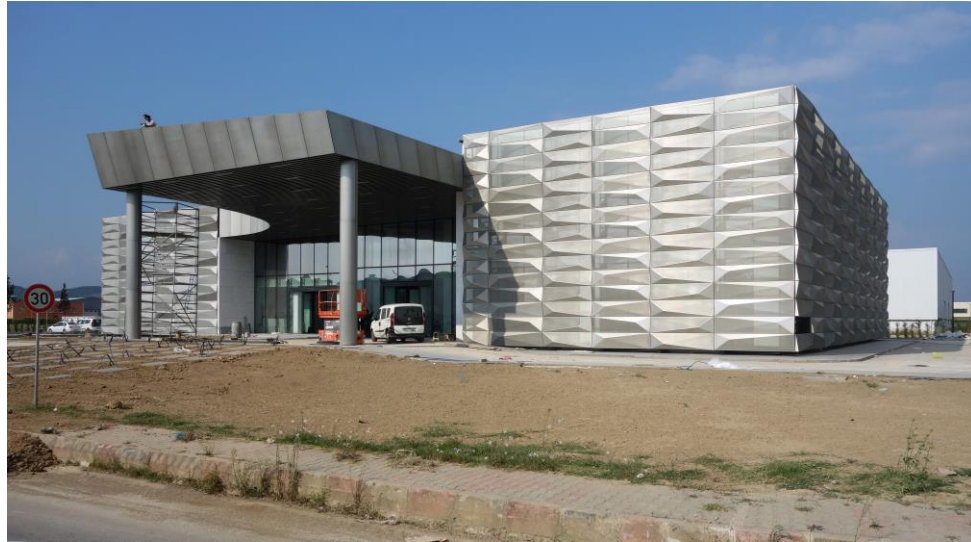
Fig. 8. Front of Sakarya Industrial Zone Headquarters and Conference Hall , Sakarya, Turkey, under construction, completion September 2016. Photo credit: BINAA.
