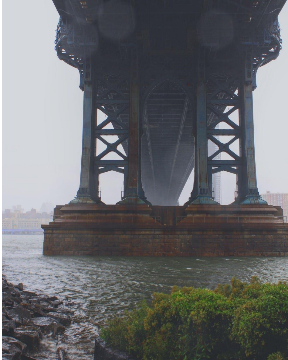
Fig. 2. Manhattan Bridge, October 2018. Down under the Manhattan Bridge on the Brooklyn side there are numerous footpaths and tidal Marshes along a path named John Street. During a driving nor'easter, I left the safety of the path and faced the tower. The conditions provided density that complements the magnificence of this 1901 structure. Photo credit: Denice Martone.
