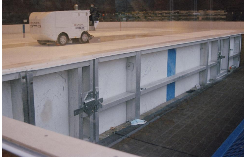
Fig. 7. Covered Rink. Lakeside, Prospect Park, Brooklyn, New York. Photograph: Khaly Durst.
