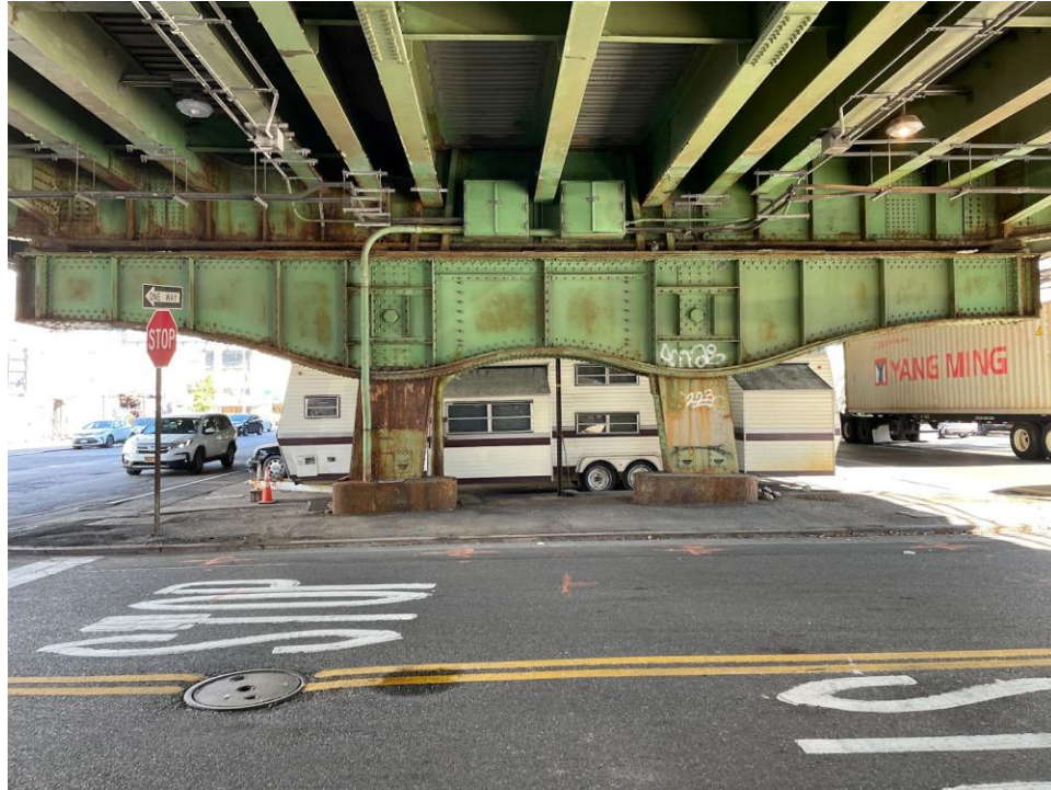
Figure 2. The Gowanus Expressway from below.
