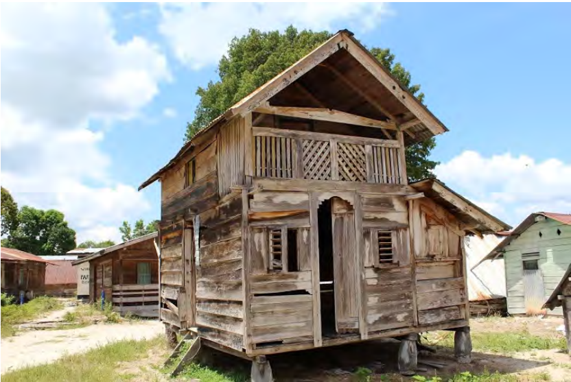
33. An older two-story home in Diitabiki constructed of local timber.
